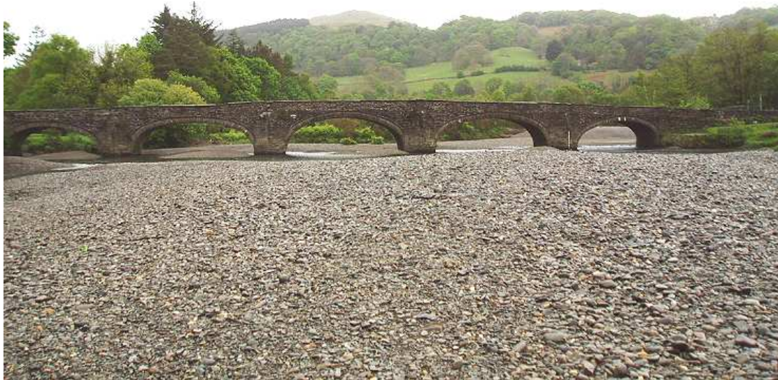
Figure 3.79: Gravel deposits around the tidal limit of the Afon Mawddach, Llanelltyd site 7
